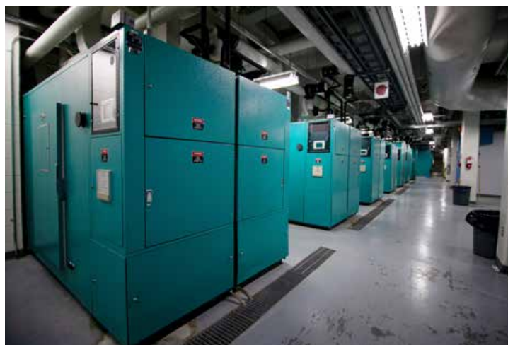
The controlled environment facility can replicate growing conditions, light intensity, temperature ranges and humidity.
